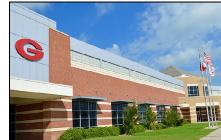
Gainesville High School Grades 9-12 | Built in 2006
