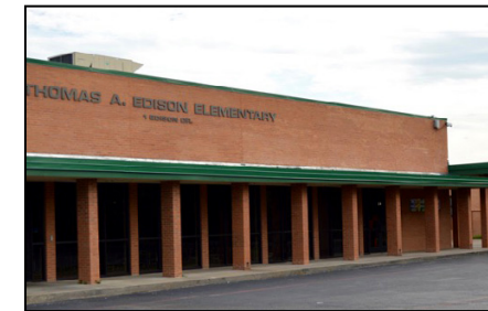
Edison Elementary Grades PreK-1 | Built in 1961
